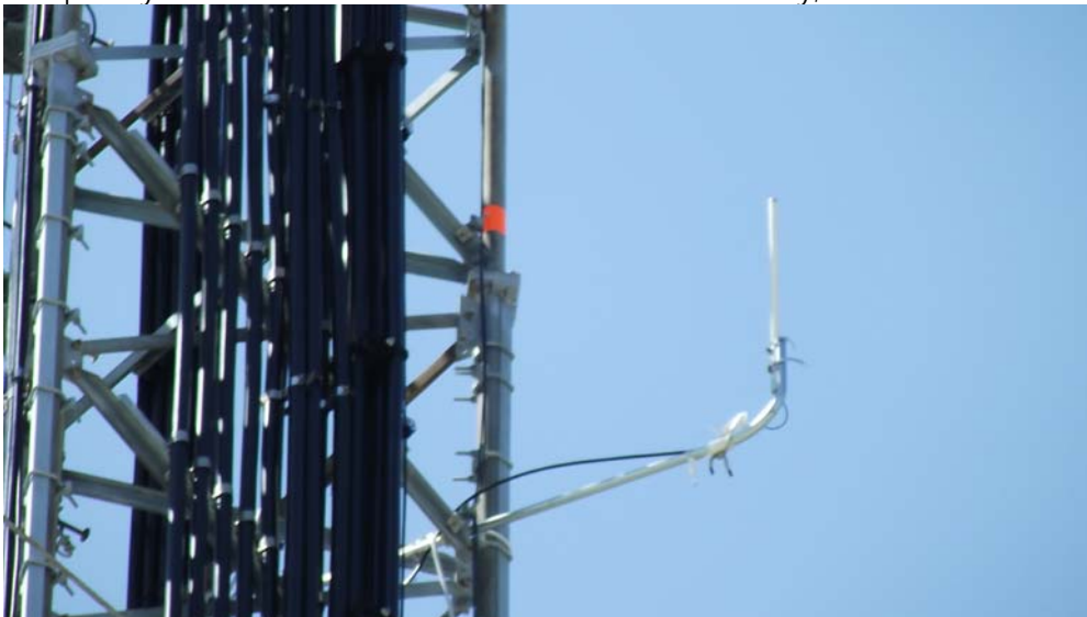
Temporary Master Radio Station Antenna for Radio Study, mounted at 100' AGL (antenna top)
